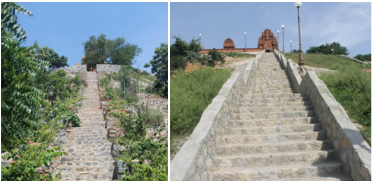
Fig. 9 & 10 The new entrance from the East offends traditional Cham beliefs about temple entrances. Source: Photo by author, 2013.
